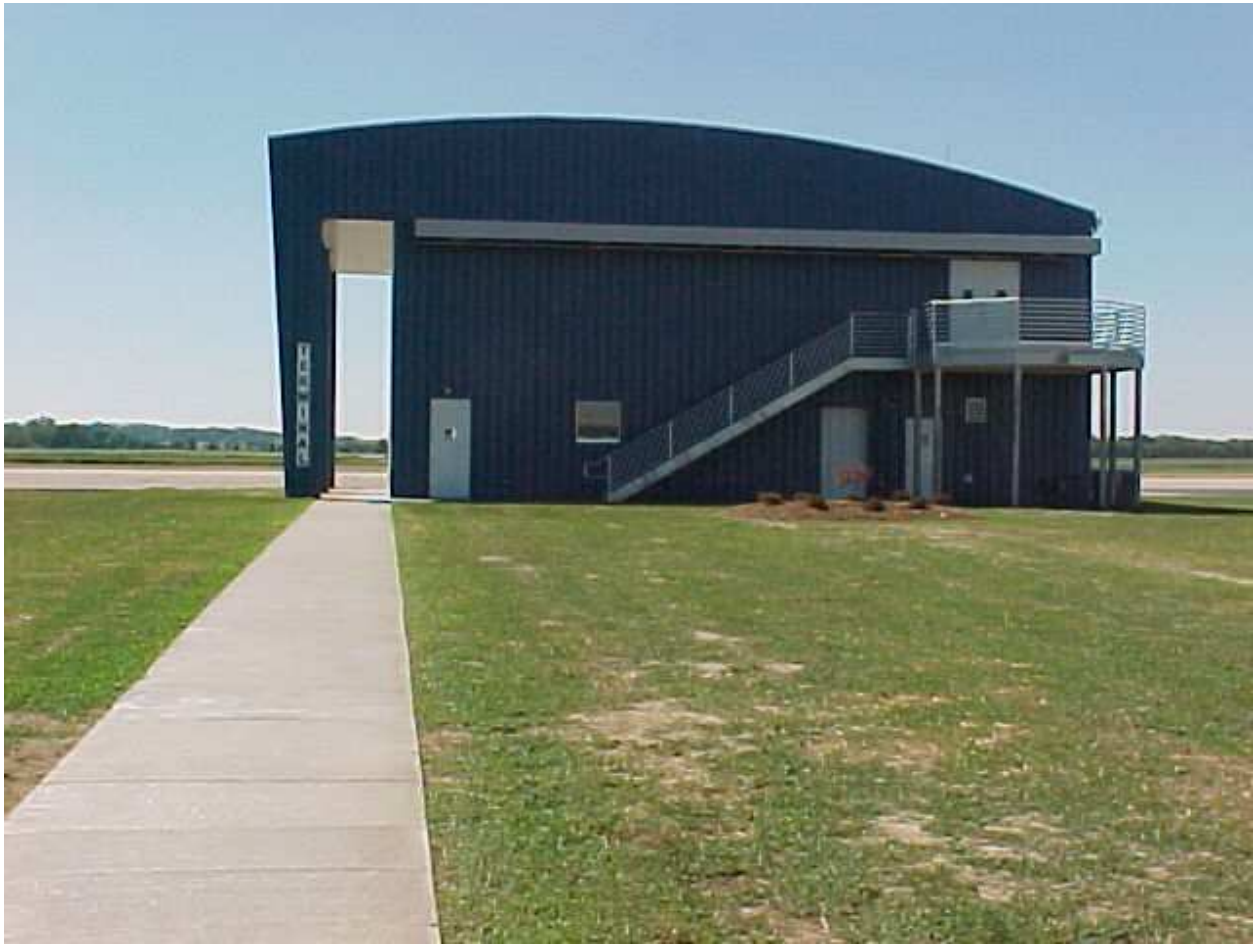
Walk-way from Public Parking to Flight Line and Terminal
